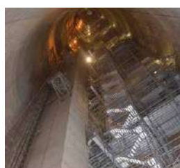
Station Thermique Noor III
